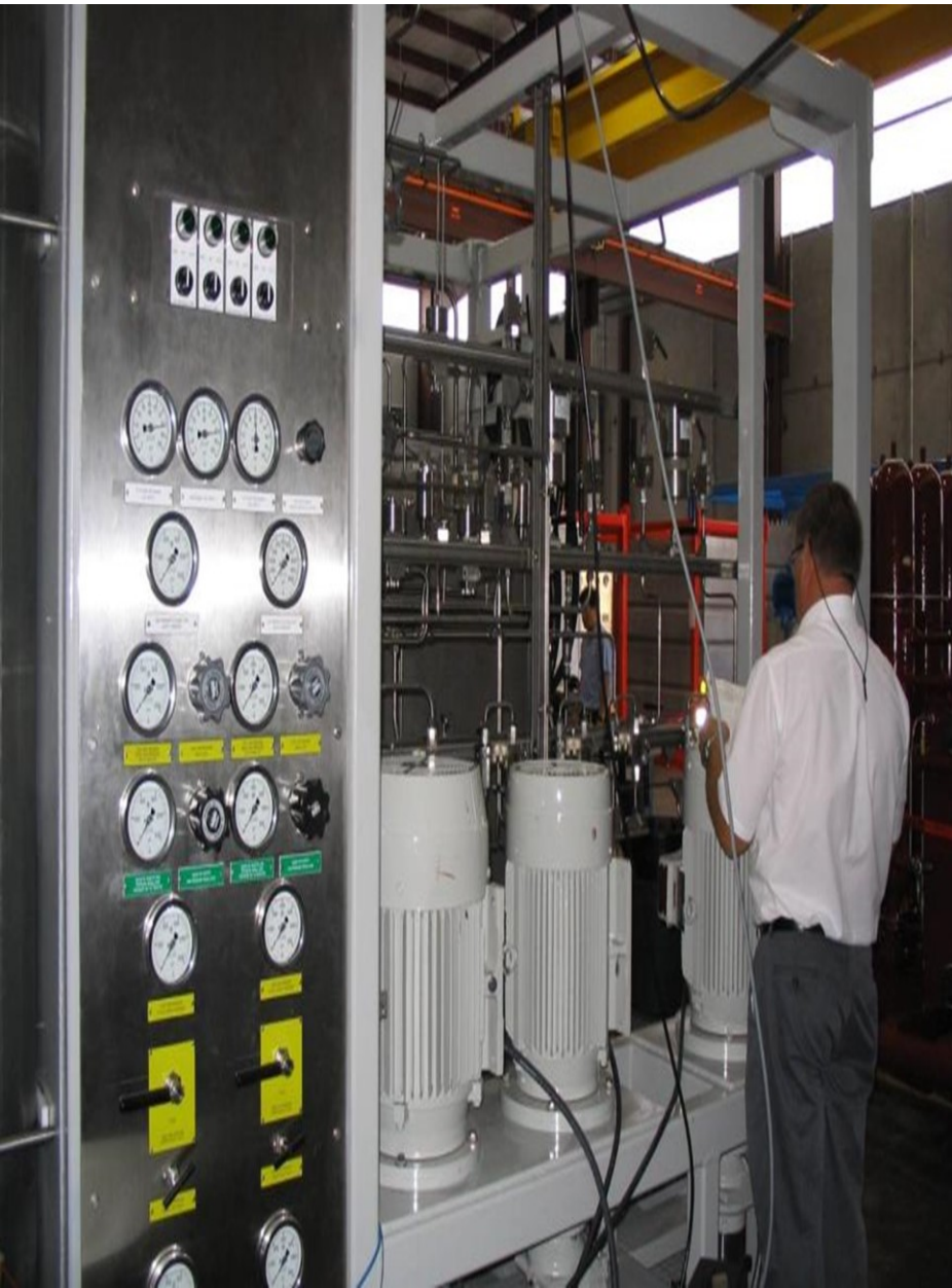
Hydraulic Power Unit
