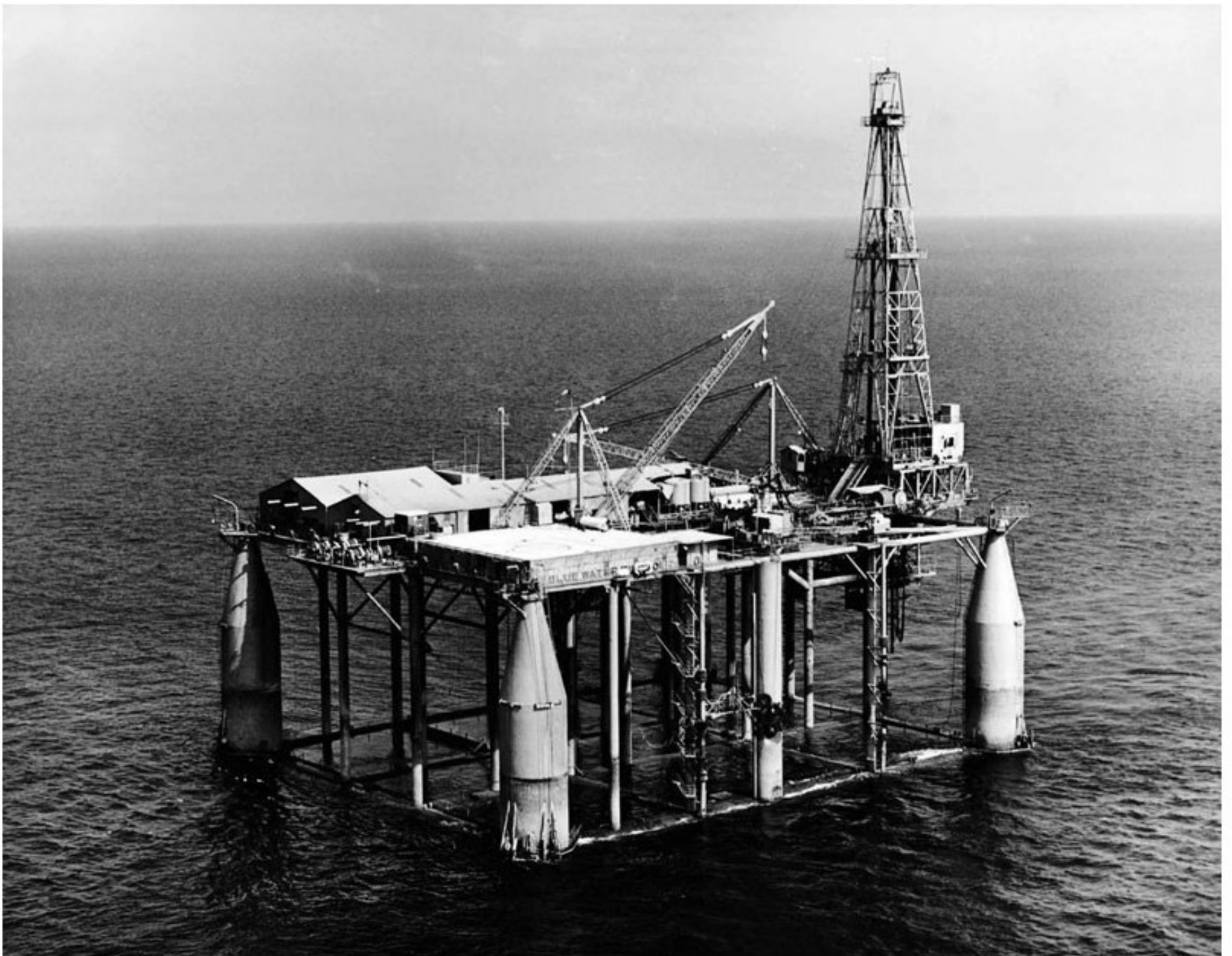
Blue Water 1 industry's first semisubmersible drilling rig 1962
