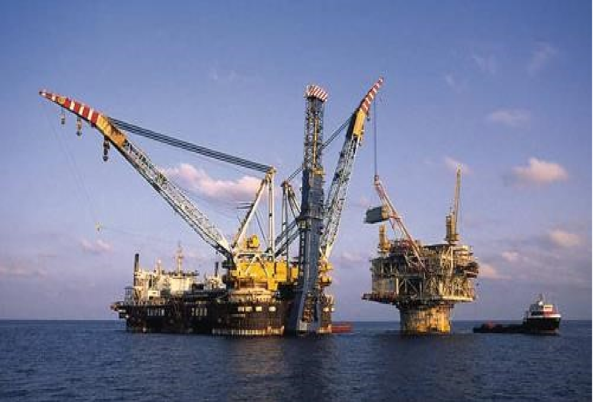
S7000 setting deck on Spar
