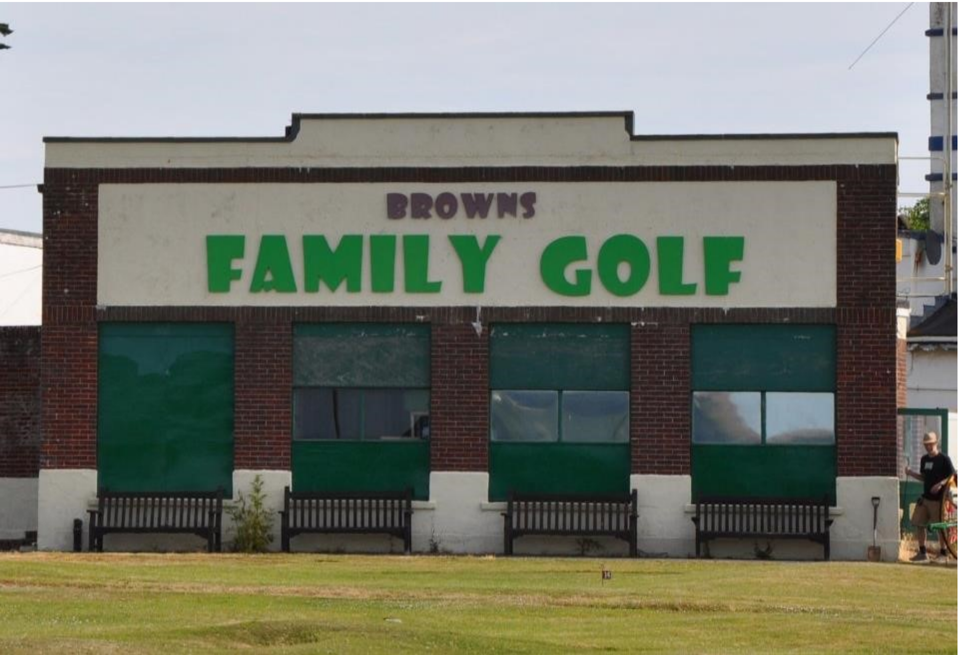
Pluto pumping station today
